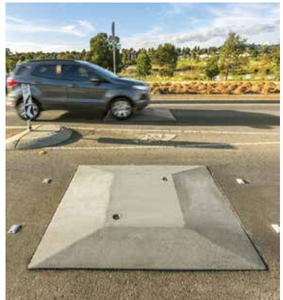
Concrete speed cushions installed in the City of Hume.
